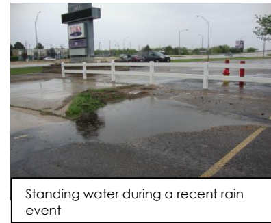
Standing water during a recent rain event
