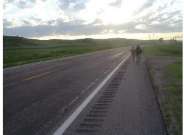
Figure 4-25 Example of Paved Shoulders
