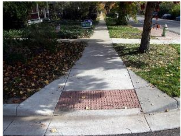
Figure 4-31 Example of Sidewalk
