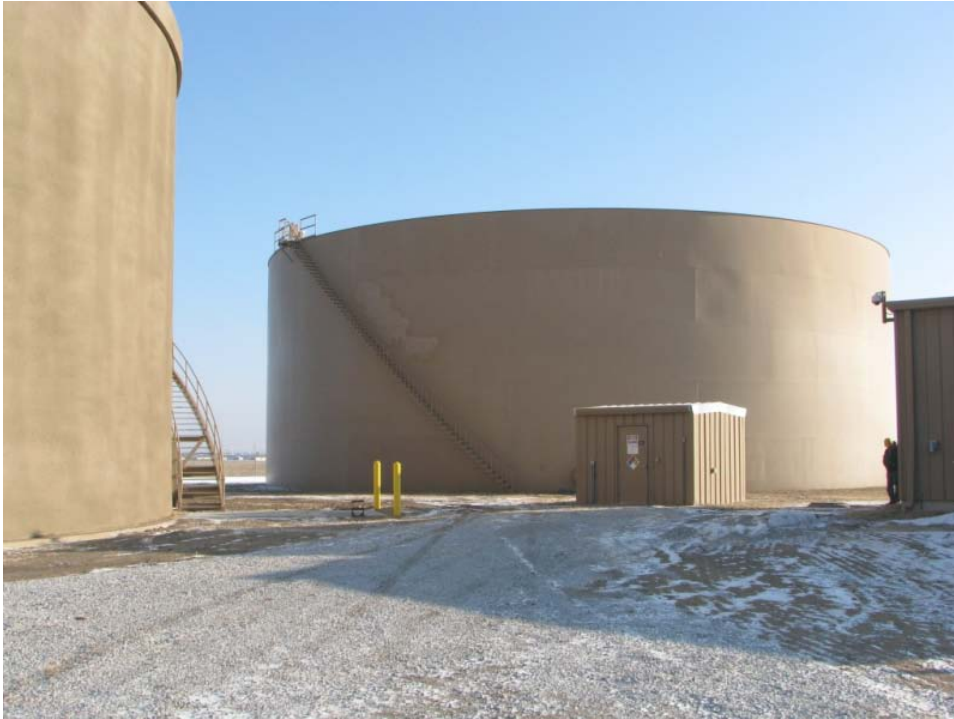
Figure 1 Rogers Reservoir 1 Pressure wash and recoat exterior.
