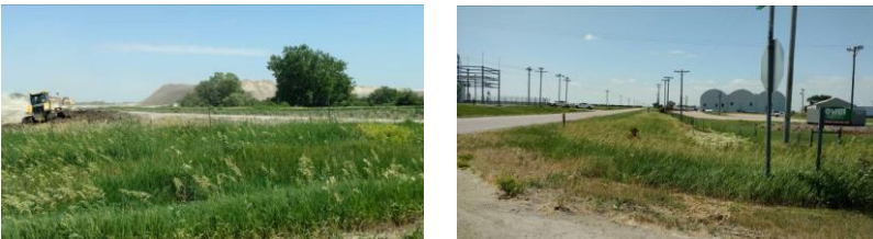
Example of the Existing Roadside Ditches
