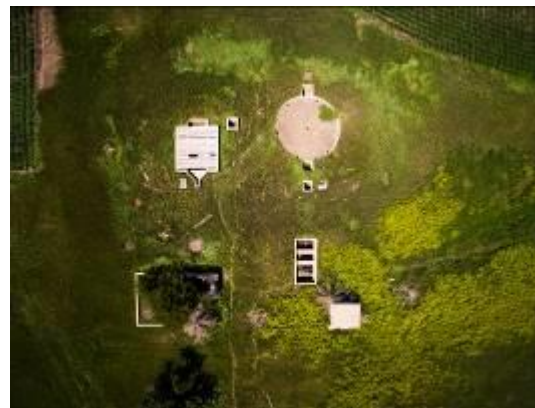
Abandoned Sewage Treatment Plant – Aerial View
