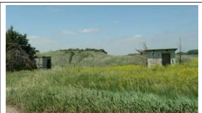
Abandoned Sewage Treatment Plant
