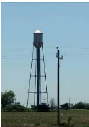
Old Water Tower located on a previously declared property (O'Neill Study)
