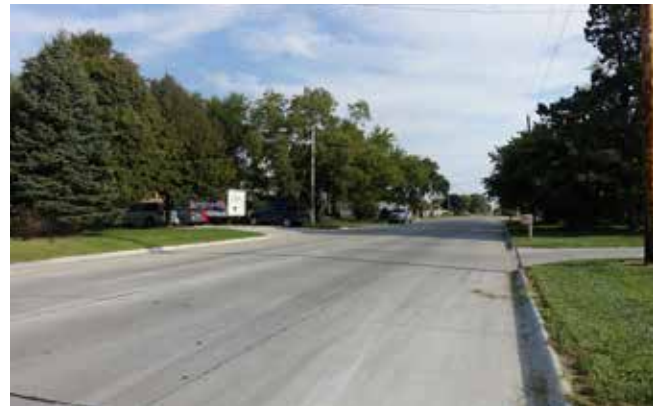
Top: Typical section of a corridor with multi-use shoulders and 2-sided parking. Above: St Paul Avenue, a potential candidate street for multi-use shoulders or striped parking shoulders.
