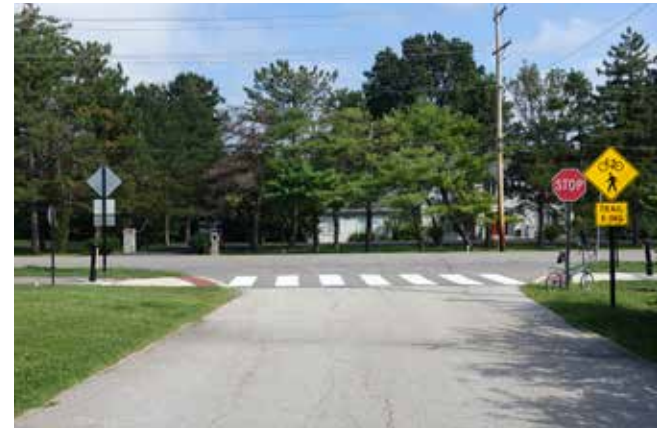
Top: Capital Avenue Trail. Above: Clayton Road sidepath in St. Louis County, Missouri. Note the highly visible crosswalk using high visibility markings and use of the trail crossing stack sign on intersecting streets.
