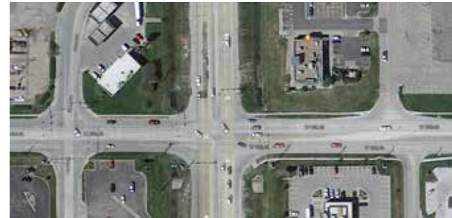
Wide corner radii create long pedestrian crossing distances. Intersections lack marked crosswalks or other crossing features such as pedestrian refuge islands (Credit: Google Maps).
