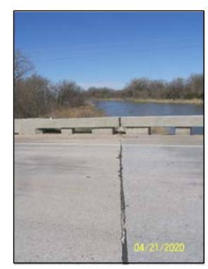
U104504125 - SOUTH - END OF FLOOR
