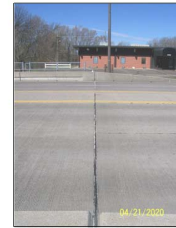
NORTH - GRADE BEAM
