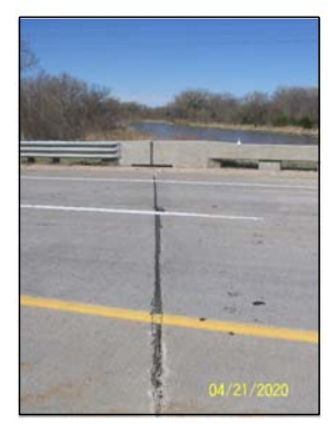
U104504125 - SOUTH - GRADE BEAM
