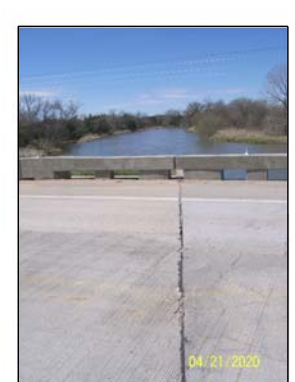
U104504120 - SOUTH - END OF FLOOR
