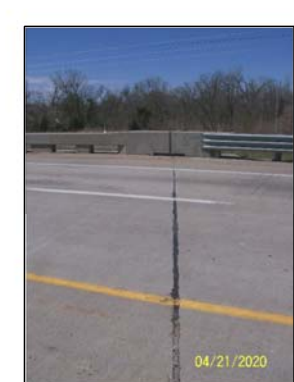
U104504120 - NORTH - GRADE BEAM
