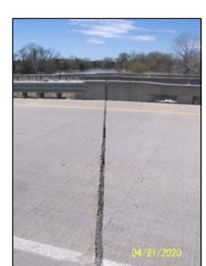
U104504120R - SOUTH - GRADE BEAM
