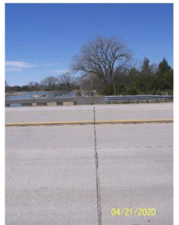
NORTH - GRADE BEAM
