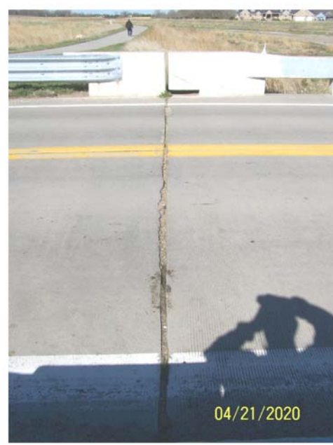
SOUTH - GRADE BEAM
