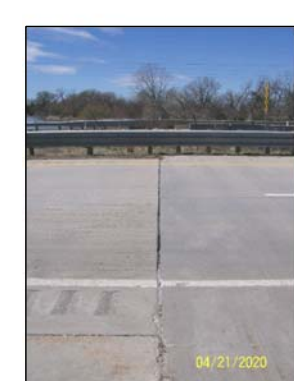
U104504120R - SOUTH - END OF PAVING
