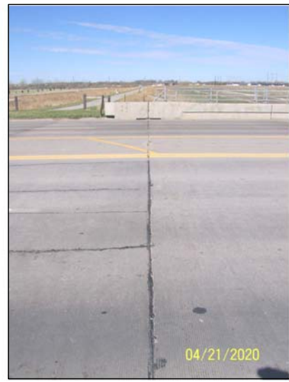
SOUTH - GRADE BEAM
