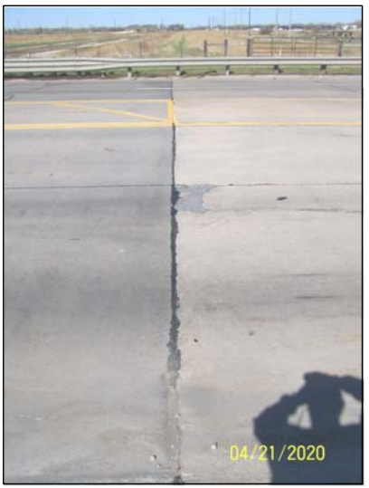
NORTH - END OF PAVING
