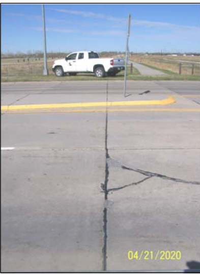
SOUTH - END OF PAVING
