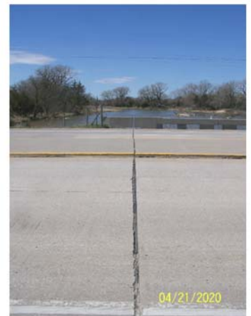
SOUTH - GRADE BEAM
