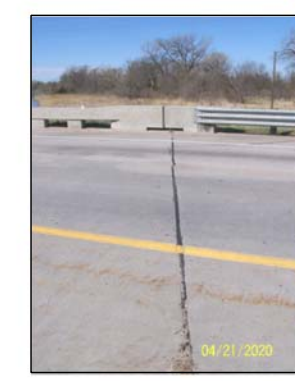
U104504125 - NORTH - GRADE BEAM
