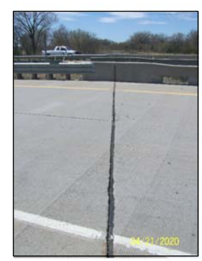
U104504125R - SOUTH - GRADE BEAM
