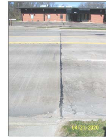
NORTH - END OF PAVING
