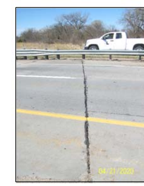
U104504125 - NORTH - END OF PAVING
