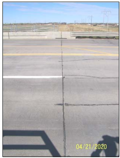
NORTH - GRADE BEAM
