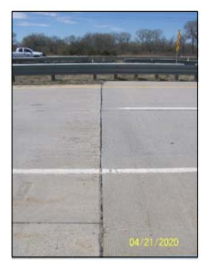
U104504125R - SOUTH - END OF PAVING
