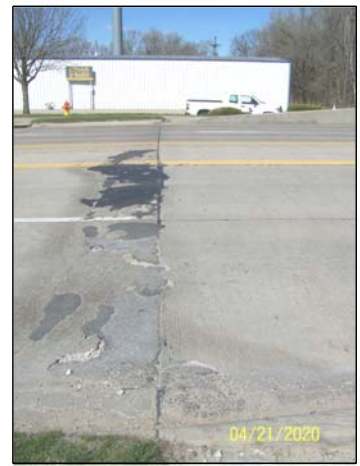
SOUTH - END OF PAVING
