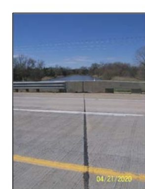
U104504120 - SOUTH - GRADE BEAM
