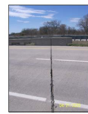
U104504125R - NORTH - GRADE BEAM
