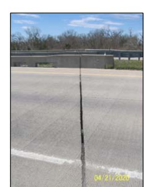
U104504120R - NORTH - GRADE BEAM
