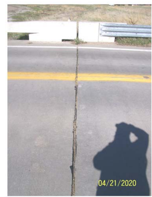
NORTH - GRADE BEAM
