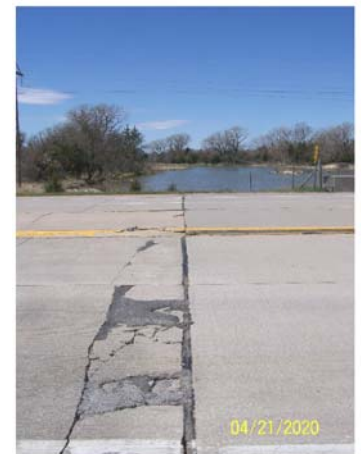
SOUTH - END OF PAVING
