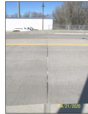
SOUTH - GRADE BEAM
