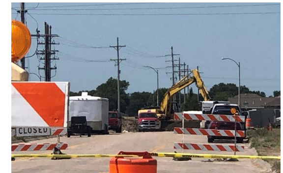
Road Construction at Faidley Ave and Claude Road, 2020
