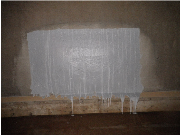
Figure 6 Rogers #2 repaired area
