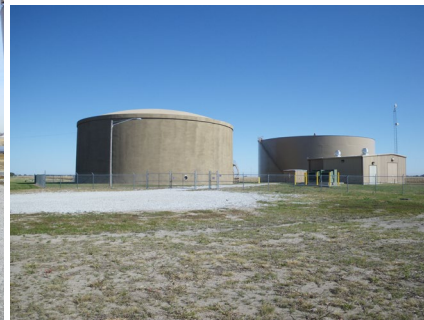
Figure 8 Rogers Pumping Station
