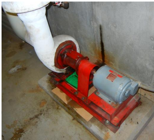
Hydronic Pump and Piping
