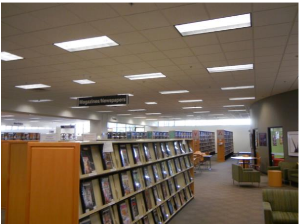
Pictures Above: Illustration of the Existing Parabolic Lighting
