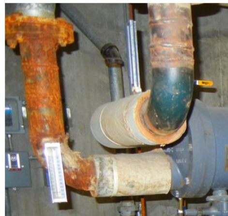
Hydronic Pump and Piping
