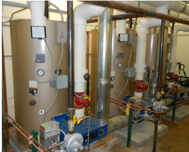
LES Fire Tube Boiler
