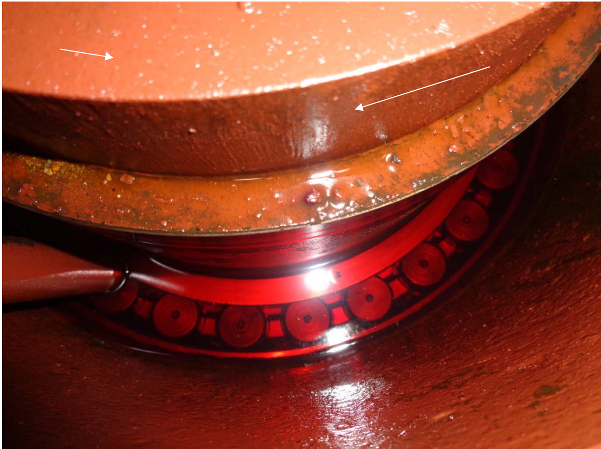
Guide bearing internals as viewed from the inspection port.
