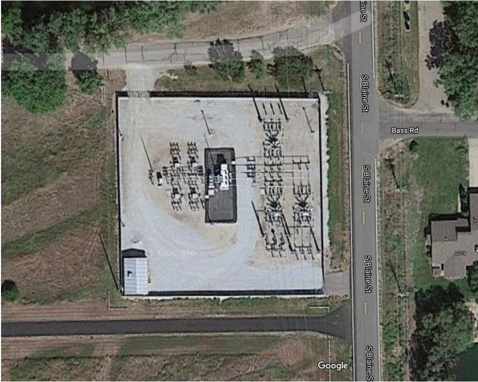
Figure 3. Substation Photographs (6 pages)
