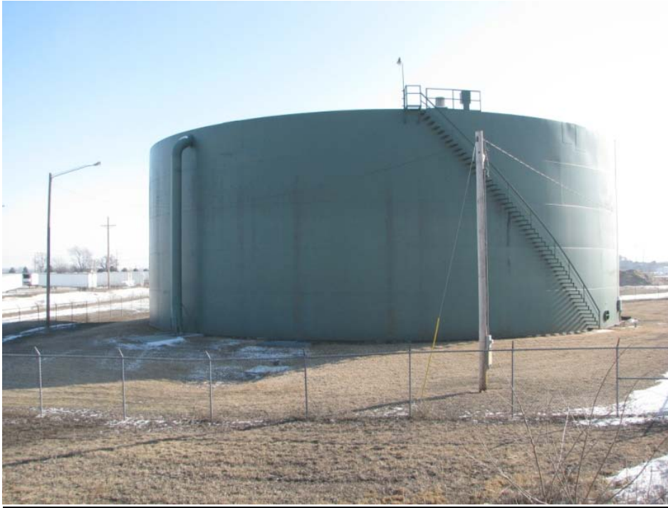
Figure 1 Burdick Reservoir Blast and recoat interior and exterior.
