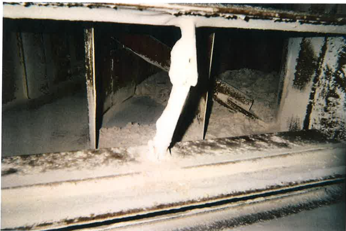
PHOTO #22 Windbox dampers.
