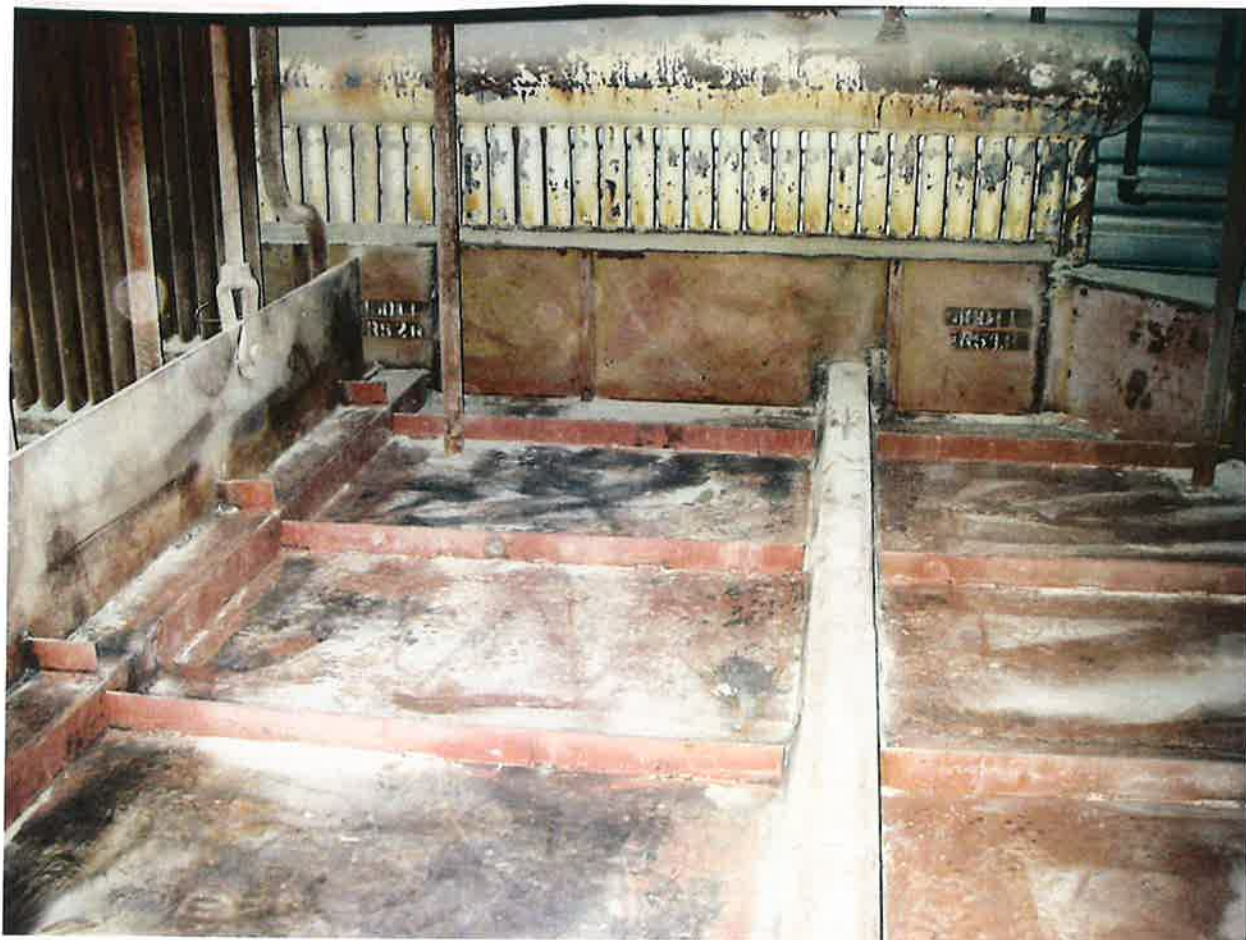
PHOTO #14 Penthouse floor casing.
