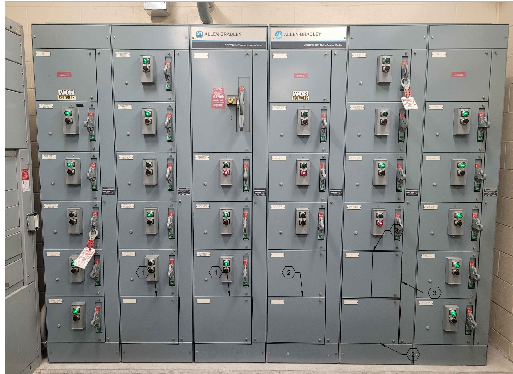
2 EXISTING MOTOR CONTROL CENTERS NO. 7 AND 8
