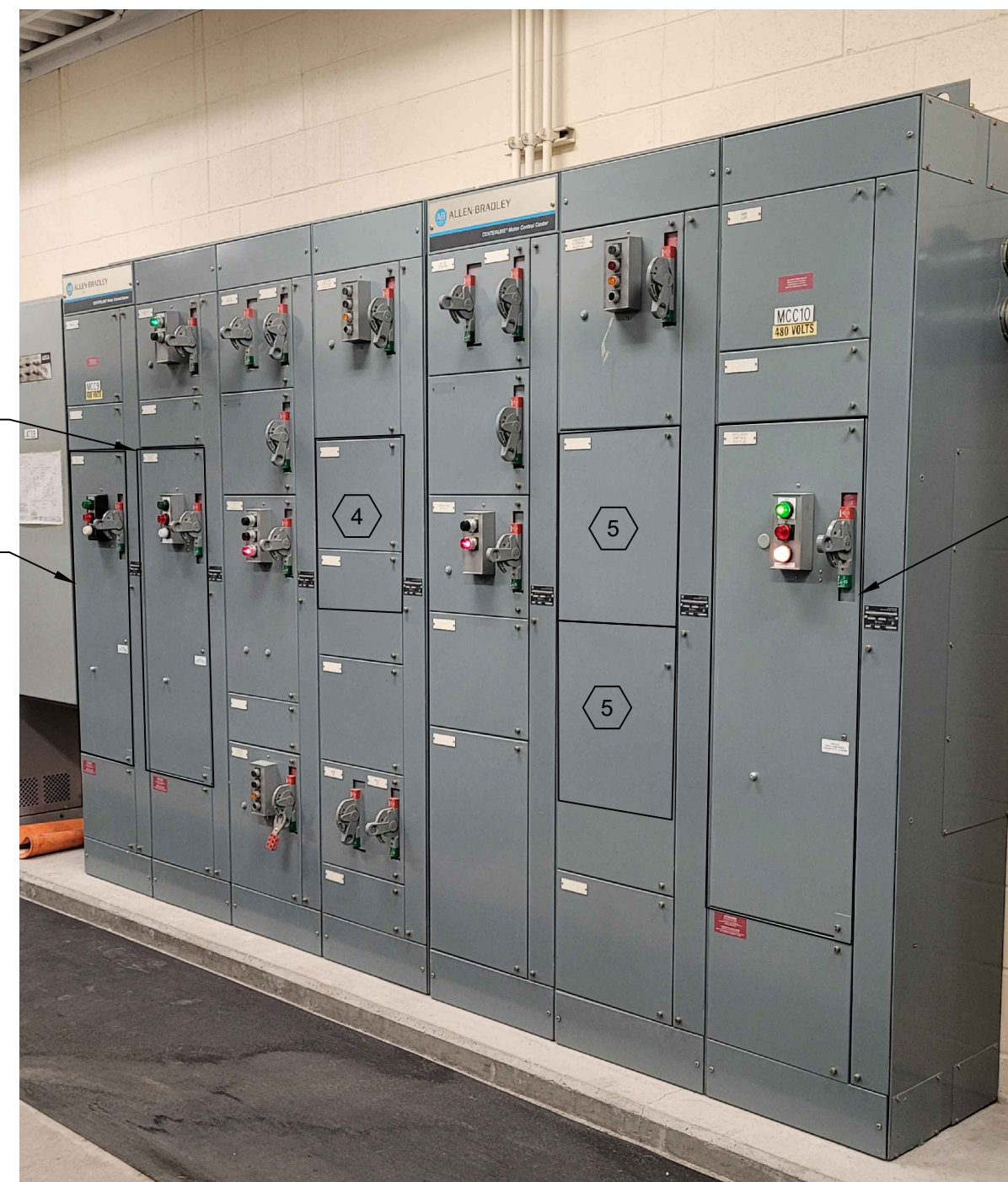
3 EXISTING MOTOR CONTROL CENTERS NO. 9 AND 10
