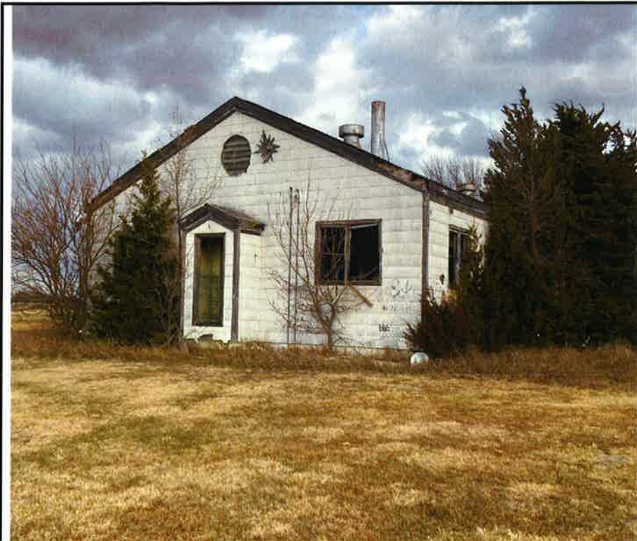
Photo 1: View of Transite siding
