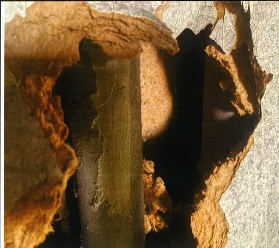
Photo 2: View of Pipe insulation.
