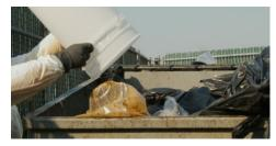
3 Dispose of the grease interceptor waste in the trash or in a designated receptacle provided by a reputable collector.
