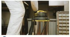
4 Pump out the settled solids and the remaining liquids.
