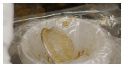
3 Remove all the accumulated grease out of the interceptor and put it in a watertight container.
