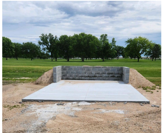
New concrete sand bunker
