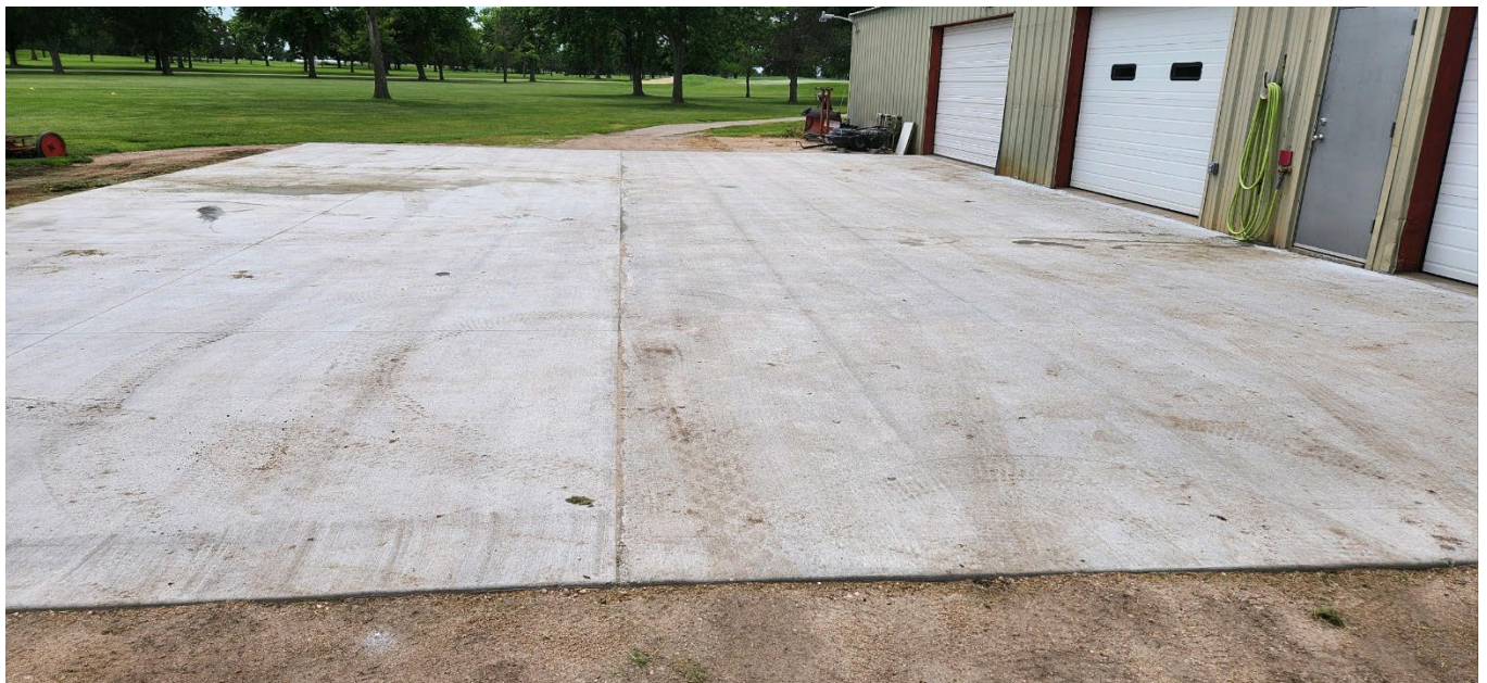
New concrete pad in front of the maintenance building
