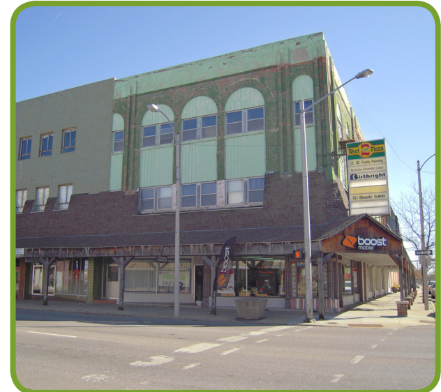
Pathfinder Building 223 W 2nd Street
