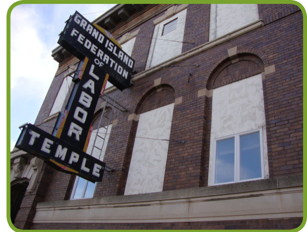
Labor Temple Building 210 N Walnut Street
