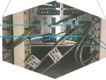
PC & DCS Connections on BN I/O Card
