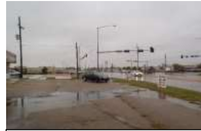
Standing water during a recent rain event
