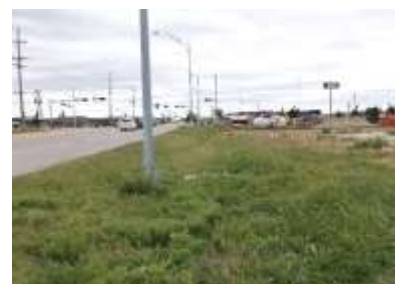
Drainage ditch along N. Webb Road
