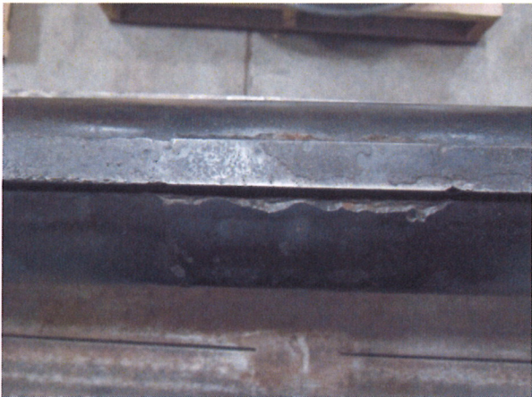
Pump shaft impeller fit & key with corrosion
