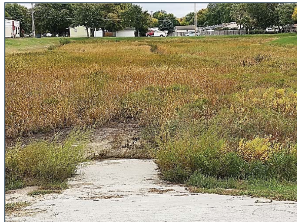
Example Vegetated Detention with no Low-Flow Liner in Commercial Development
