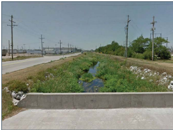
Examples of Existing Area Vegetated Treatment Ditches
